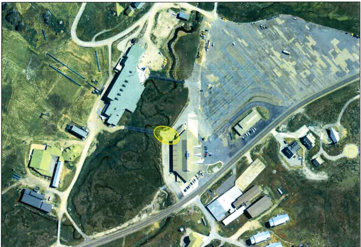
Figure 1: Location of works in context of Skitube Terminal, Perisher Car Park and Front Valley ski area (Source: SIX Maps 2016).
